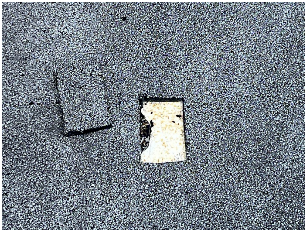
Section D: Test Cut # 1 – Dry
