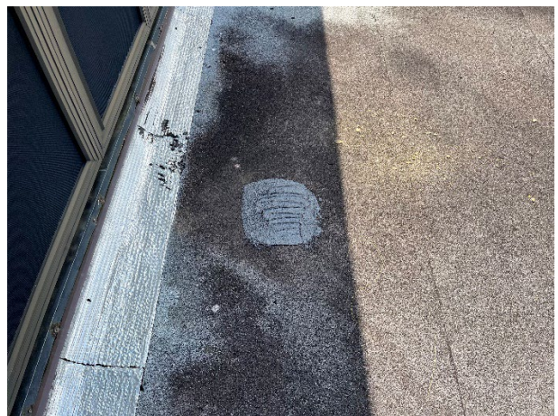
Section F: Test Cut repair patch
