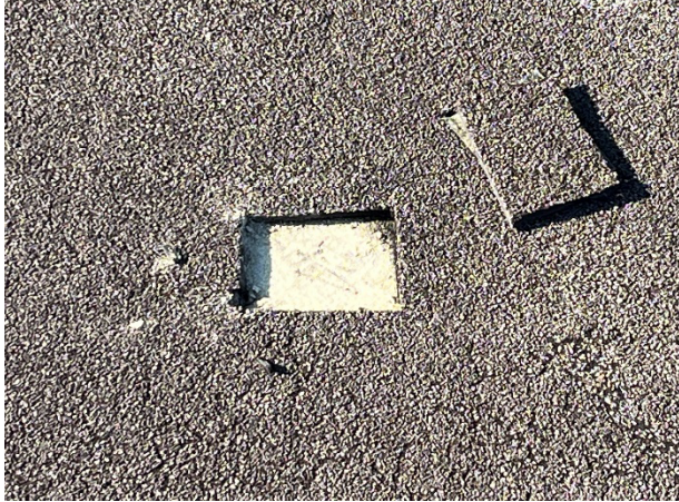
Section B: Test Cut – Dry
