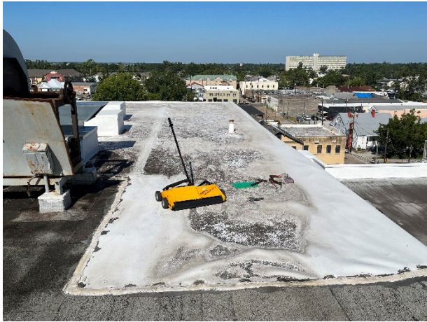
Section A: temp single-ply membrane installed
