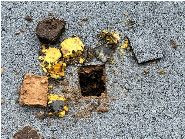
Section E: Test Cut # 1: Saturated
