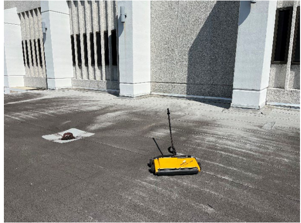
Section C: No moisture detected in this roof section
